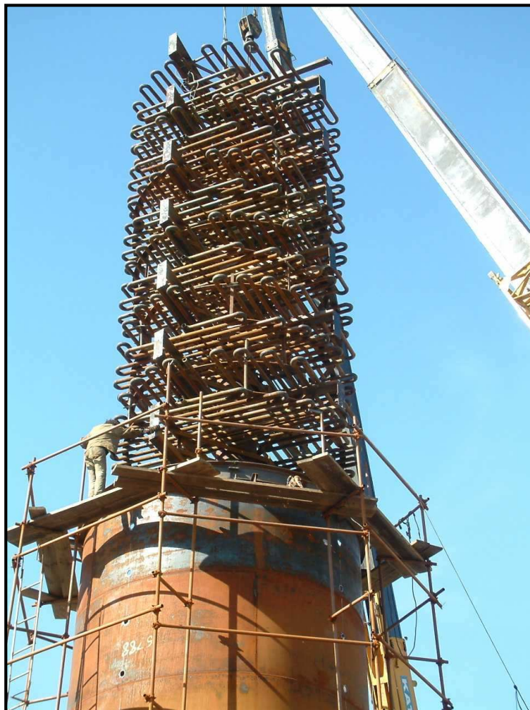
Figure 4. A cooling element and stirrer assembly being fitted into a VC shell.
